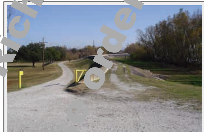
Riverfront at Chalmette Battlefield in St. Bernard Parish: crest of natural levee on left; artificial levee with floodwall at center; willow-covered batture at right. The Mississippi flows about 150 feet beyond the batture. Photograph by author, 2003.
