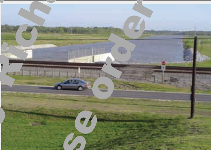
Seen here is Davis Pond’s intake in the Mississippi River (left) and outflow canal into the swamp near Luling, twenty-two miles above New Orleans. The diversion, opened in 2002, releases up to 10,650 CFS of river water into 777,000 acres of Barataria Basin marshes. It is often called the largest coastal restoration project in the world. Photographs by author, 2004.
